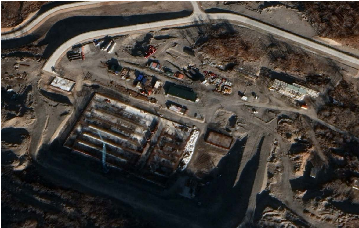
Figure 6: New nuclear warhead storage under construction. Source: Google Earth.
